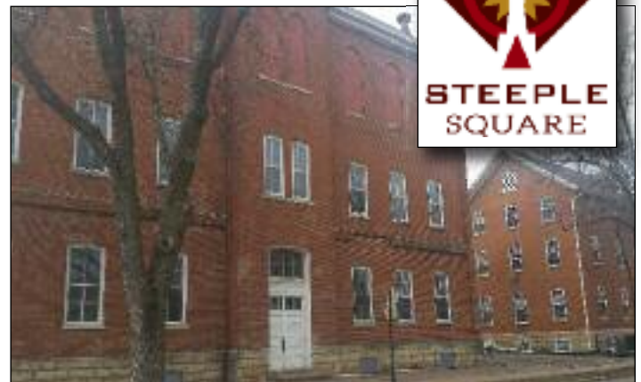
The former Jackson School is located just south of the Maria House. Construction to transform this building into 12 apartments will begin this May. For more information on the Steeple Square project, visit www.steeple-square.org .
